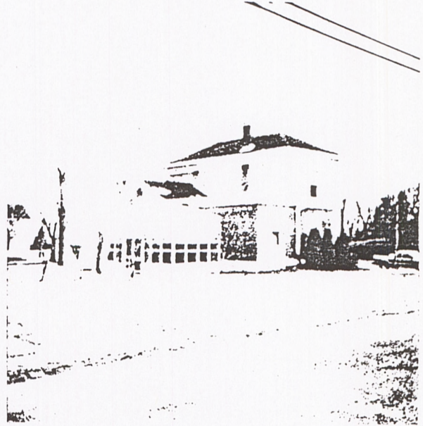
2. Needs new roof and brick tuck. New foundation is needed due to walls pushing in.
