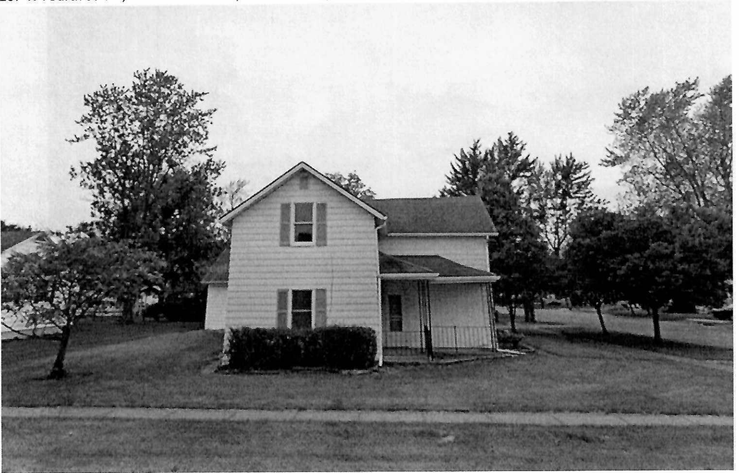
249 W Canal Street; foundation bad, needs new windows, siding, porch collapsing; or needs torn down
